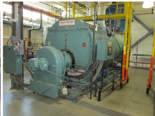
Figure 6005.6 Typical Steam Boiler
