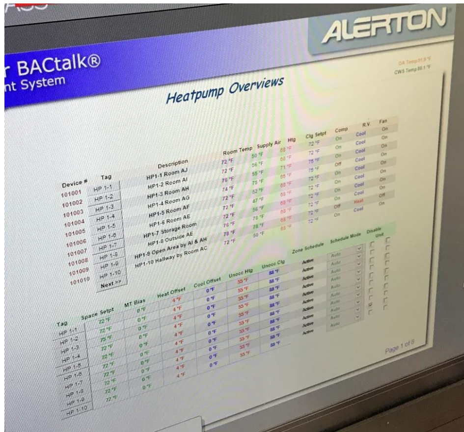
Figure 6018.5 BAS Screenshot Showing Temperature Setpoints for Each HVAC Unit
