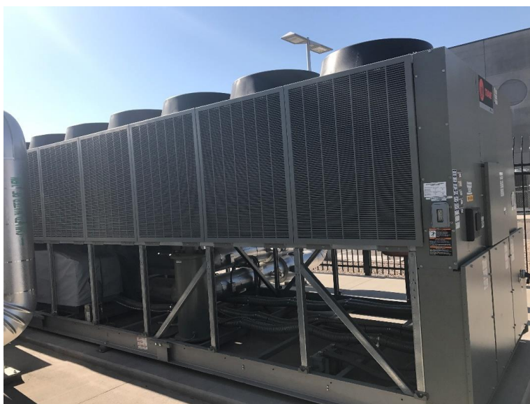
Figure 6007.3 Typical Air-Cooled Chiller
