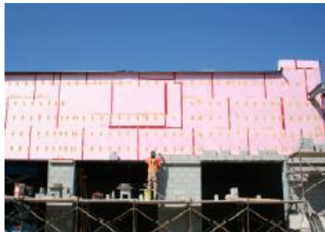
Figure 5018.2 Example of Cavity Insulation 1 Figure 5018.3 Example of Continuous Insulation 2
